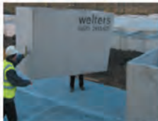
Burial Chamber Installation in saturated land
