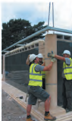
Circular column installation
