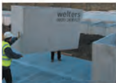
Burial Chamber Installation in saturated land
