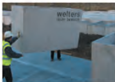
Burial Chamber Installation in saturated land
