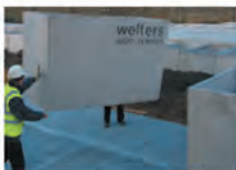
Burial Chamber Installation in saturated land
