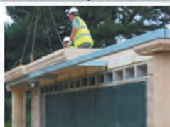
Specially design roof panel section installation
